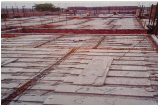
Figure 01: Plank and Joist roof
