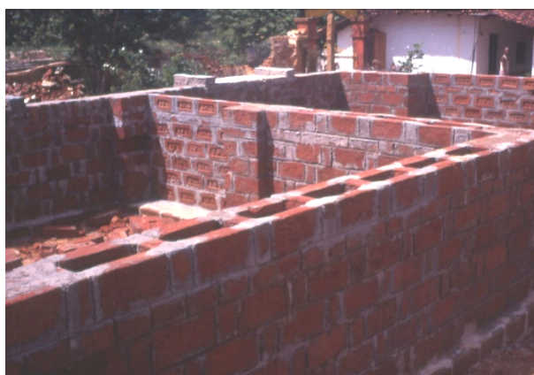
Figure 01: Wall construction with rat-trap bonds
