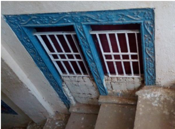
Figure 22: View of room window opening into the access staircase
