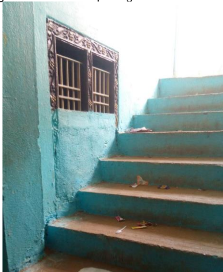
Figure 38: Window opening onto the staircase
